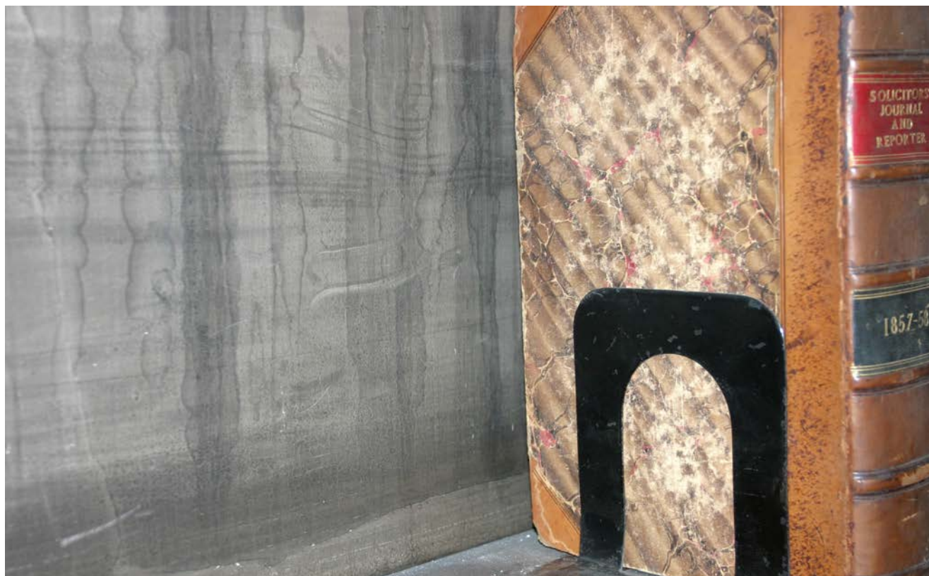
This wall in the State Library of Iowa—Law Library still shows heat, smoke, and possibly water damage.
