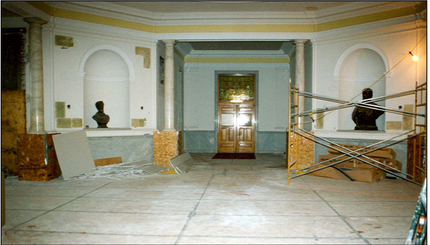
Renovation is in progress on the first floor looking west. 1997
