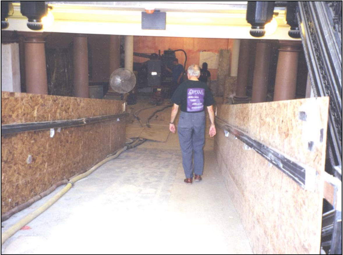
Ramp over stairs from back, 1999
