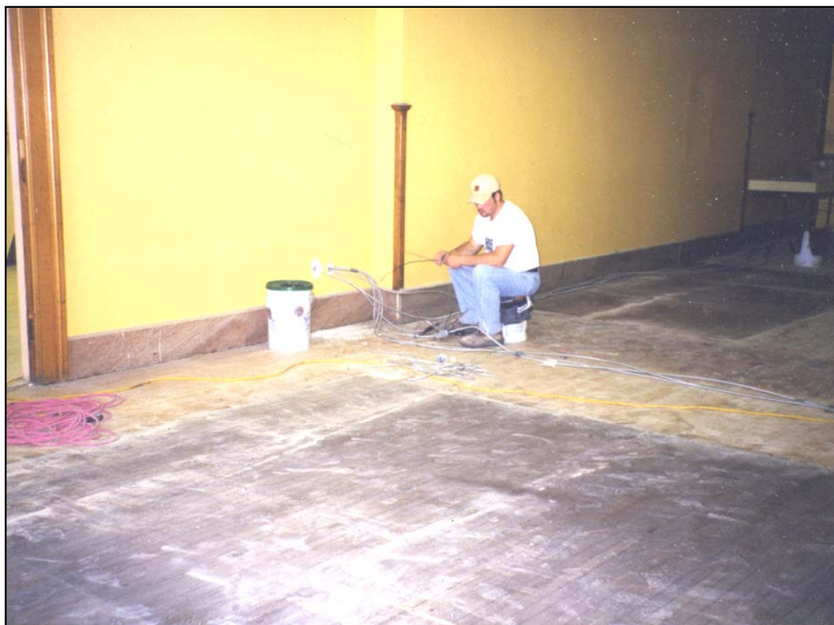
An electrician installs new wiring. 1999
