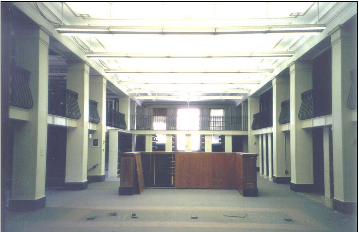
The main library on the first floor is shown during renovation. 1997
