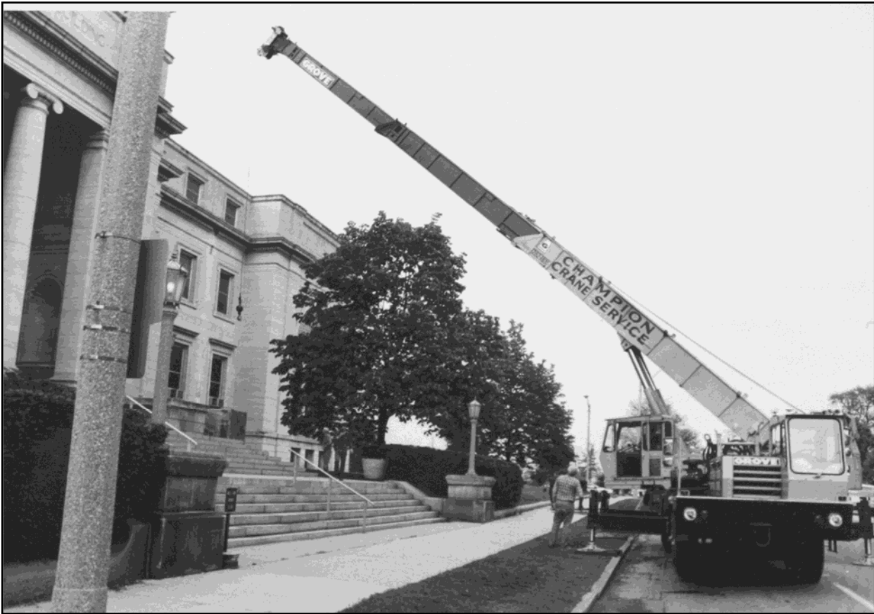
Installation of a new electricity transformer, 1984
