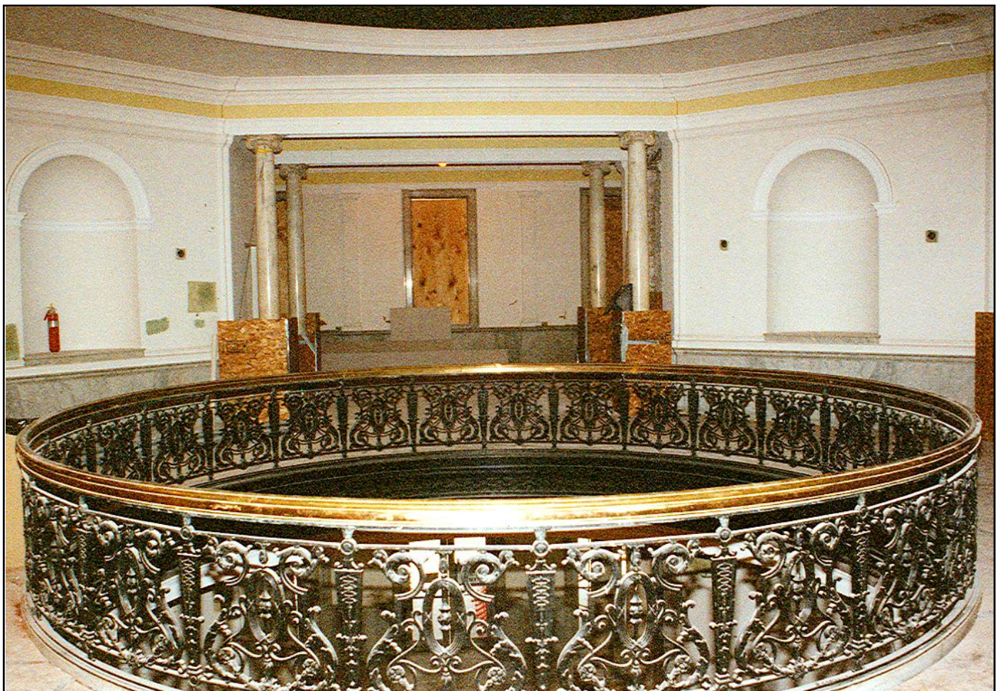
The second floor rotunda during renovation, 1997
