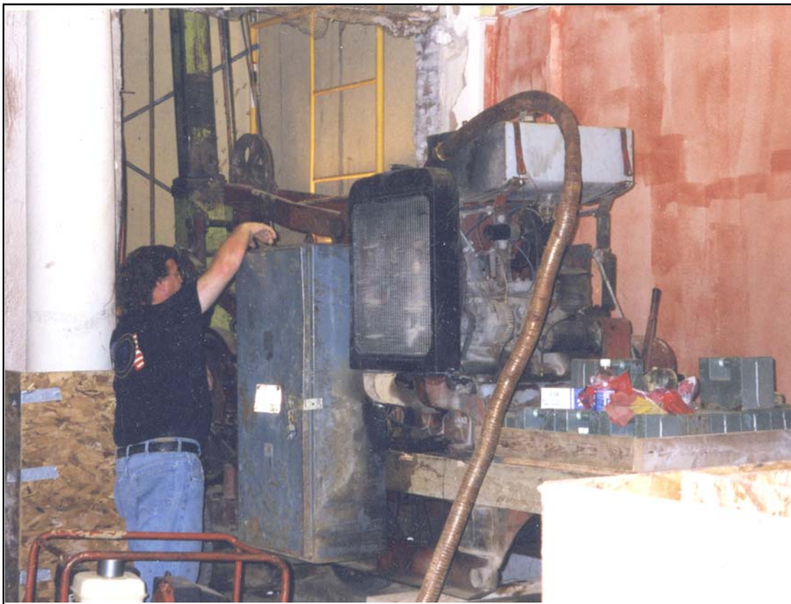
Elevator installation, ground floor, 1999
